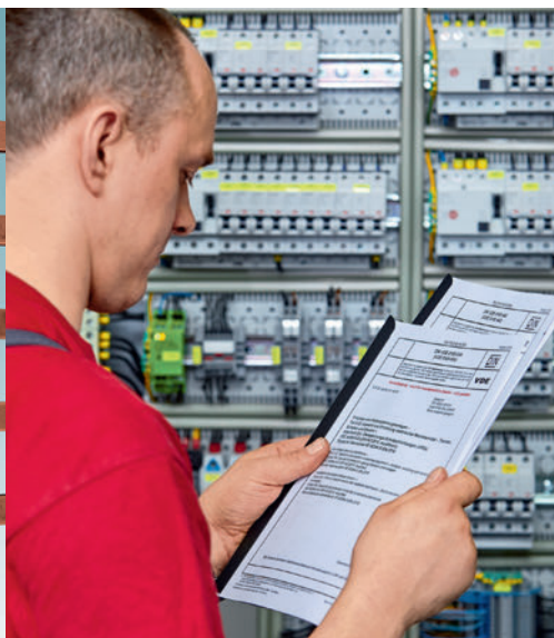
The best place for surge protection is directly in the main distribution board.
